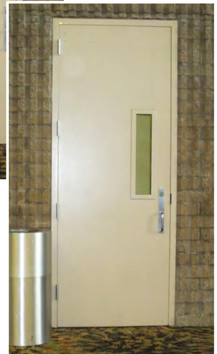
vision lite or sidelite, the 2010 ADA standards and ICC A117.1 both require the bottom of at least one lite to be no more than 43 inches above the floor. This is new to the ADA standards but has been required by ICC A117.1 for decades.
