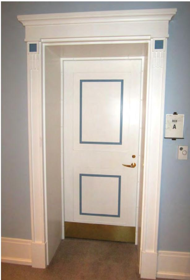
**A door in an alcove or a frame with a large jamb depth can trigger a requirement for extra maneuvering clearance at the door leaf.**
