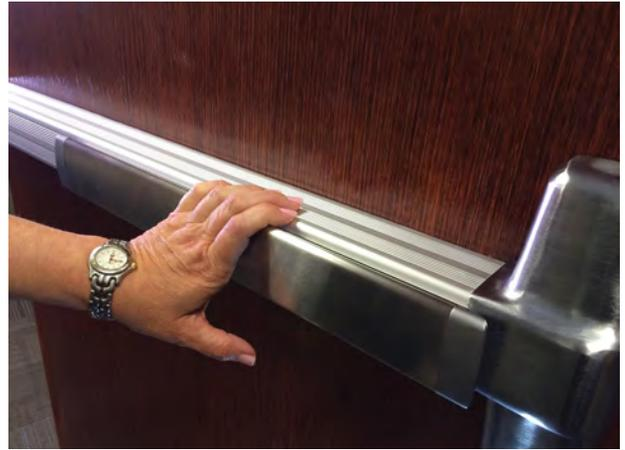
**Panic hardware has traditionally been required to operate with no more than 15 pounds of force. New ADA requirements limit the operation of door hardware to a maximum of 5 pounds.**
