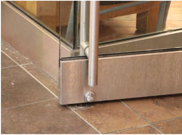
**Protruding hardware within the bottom 10 inches of a door could inhibit passage through a door opening by catching a crutch, cane, walker or wheelchair.**
